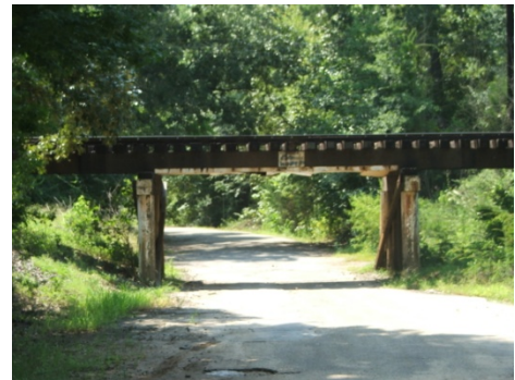
Railroad truss over entry road
