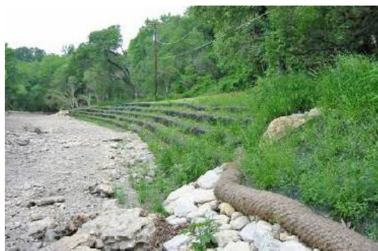
Bioengineering: mechanically-stabilized earth and plantings.
