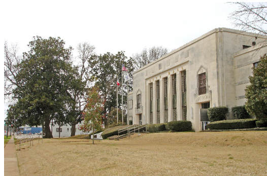
City Hall needs many interior upgrades, but renovations should preserve the building's historic character.
