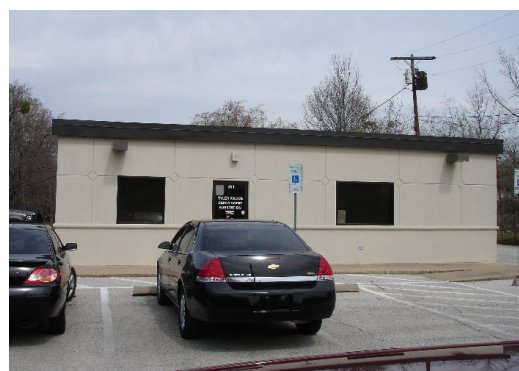
North Tyler police substation
