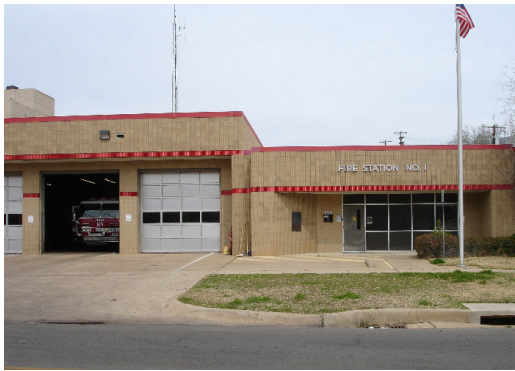
Fire Station No.1 in downtown Tyler
