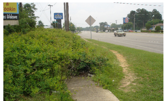
Dead-end sidewalk and a “desire line” showing that pedestrians need a continuation of the sidewalk.
