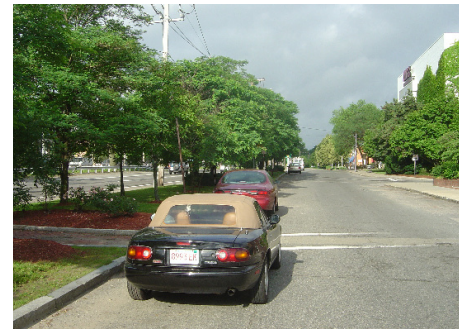
Local access drives separate cars going to businesses along arterials from through traffic.
