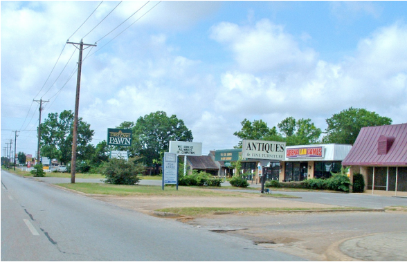
Numerous curb cuts/driveways within short distances of each other create traffic congestion on arterials.
