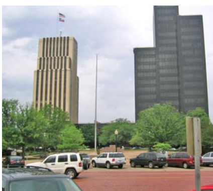
Office towers on each end of the west block of the square leave an awkward empty space between them.
