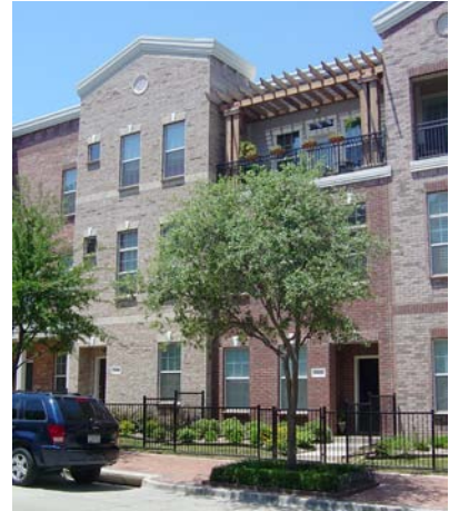
Townhouses, Addison Circle (TX)
