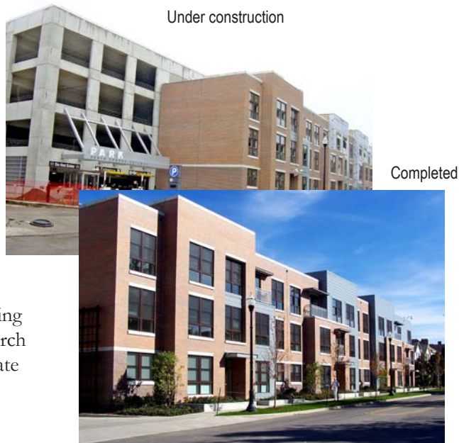
Townhouses can line the edges of parking garages and create an attractive street environment.
