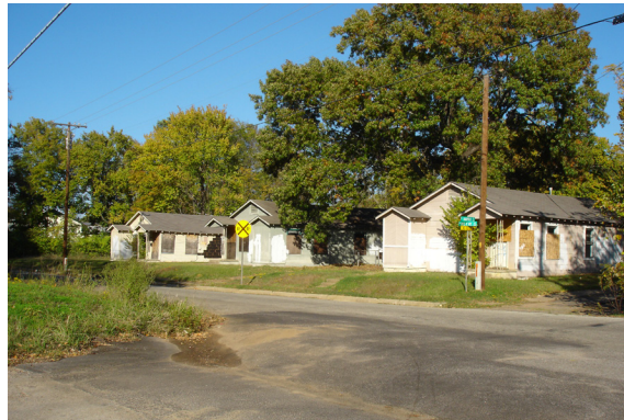
Boarded-up buildings can destabilize neighborhoods and discourage new investment.
