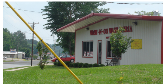
The windows, door, roof overhang and lettering in a simple contrast trim color help this metal building make a better impression.
