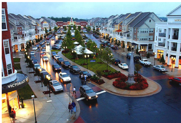
Birkdale Village in Huntersville, NC is a mixed-use development with most of the housing units above village-style retail. (Source: ULI Case Studies)
