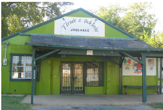
A simple paint scheme can make a metal building more attractive, like this one in Tyler.
