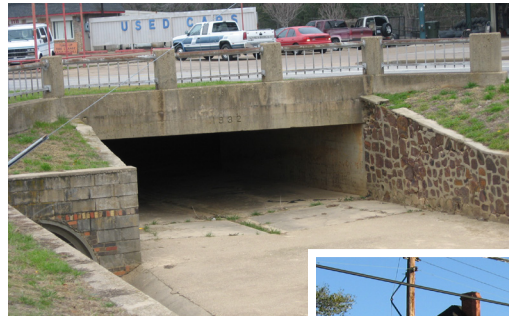
WPA drainage canal (1932)
