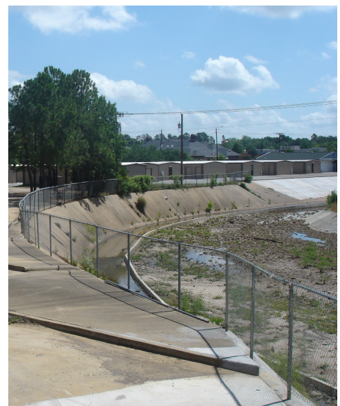
Concrete-lined drainage canals improved with trees and plantings can reduce heat effects, help with stormwater filtration, and provide wildlife habitat.
