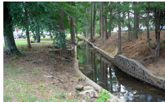
WPA drainage canal
