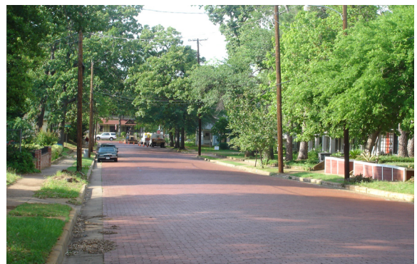
Chilton Avenue in the Brick Streets National Register Historic District
