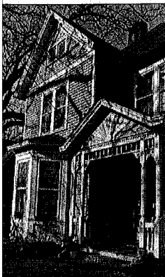
Wood spindles and columns, pierced brackets, and a herring pattern of flush boards in the porch gable of this 19th-century house illustrate the versatility of wood for detailing.
