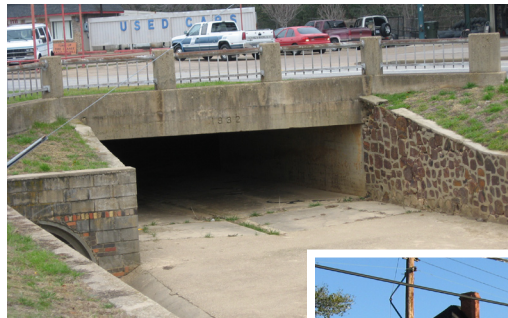
WPA drainage canal (1932)
