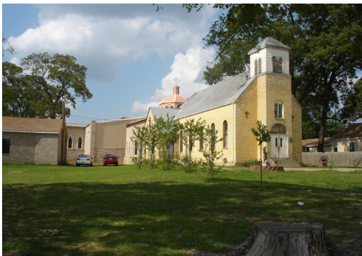
St. Peter Claver Catholic Church, North Tenneha Avenue
