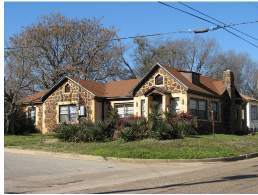
Stone house in North Tyler
