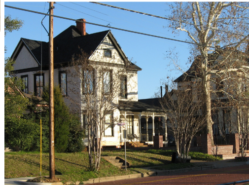
Victorian-era homes on South Fannin Avenue
