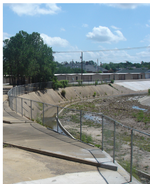
Concrete-lined drainage canals improved with trees and plantings can reduce heat effects, help with stormwater filtration, and provide wildlife habitat.
