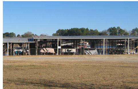
In addition to supplying drinking water to the city, Lake Tyler provides recreation amenities, such as boat ramps (top) and boat stalls (bottom).
