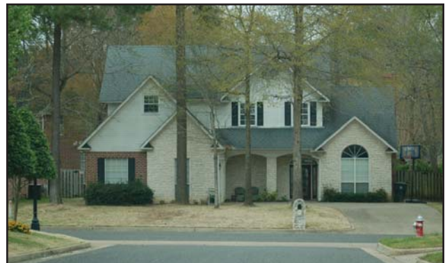
Typical single-family home in The Woods subdivision
