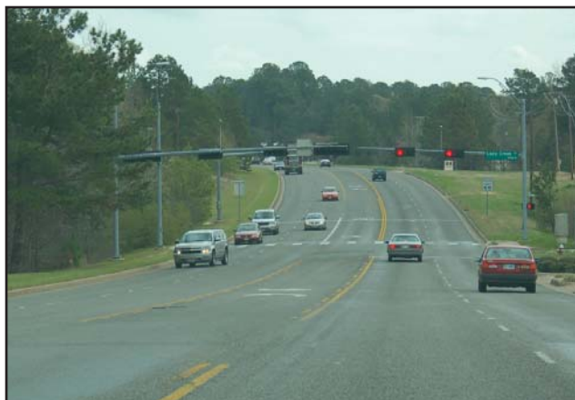
Disconnected Lazy Creek Drive intersection
