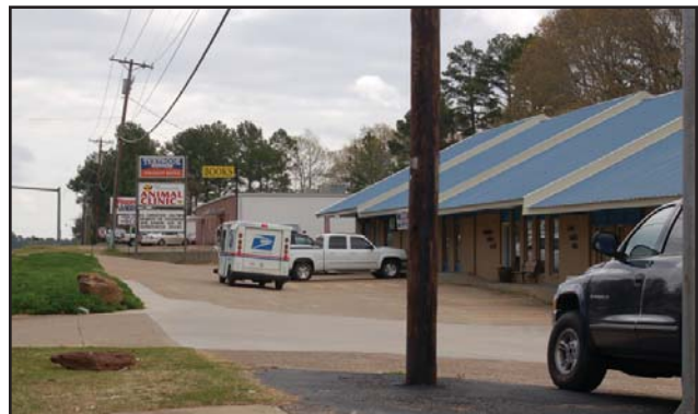
Typical study area commercial buildings
